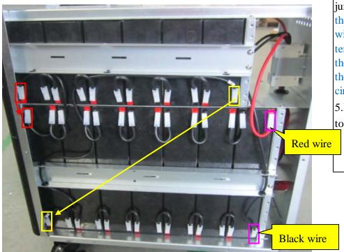
4. As picture: insert the battery jump wire. Notice: while insert the battery wires, make sure the wires are not damaged, the terminal should be inserted well, the pliers should keep away from the battery terminal, avoid short circuit.
